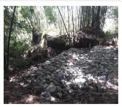
Figure 15: The embanlment of the rivulet using gabon wire and stone in Simariya Tole.
