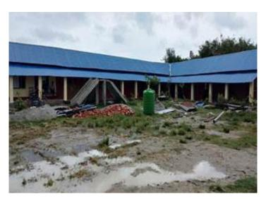
Figure 2 : CGI sheets supported to as a part of the mitigation work identified from the prepared LDCRP of the particular ward at Mahendra school Gramthan, Morang
